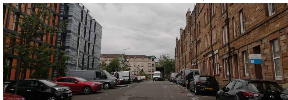
6. Gibson Street, mix of building typologies.
